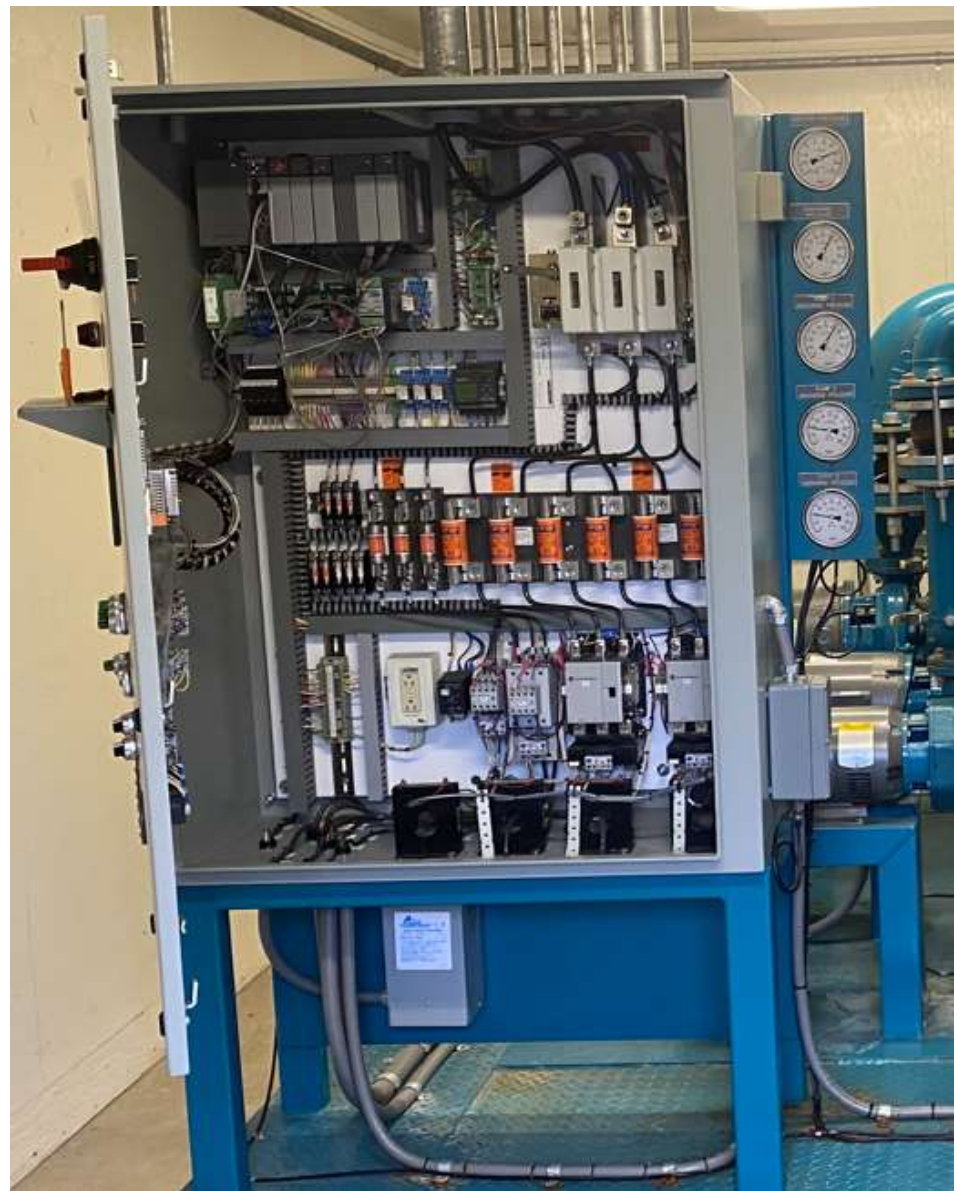
Existing Pump Control Panel: Replace internal backpanel assembly complete. Remove existing door devices and replace with new door skin and devices.
