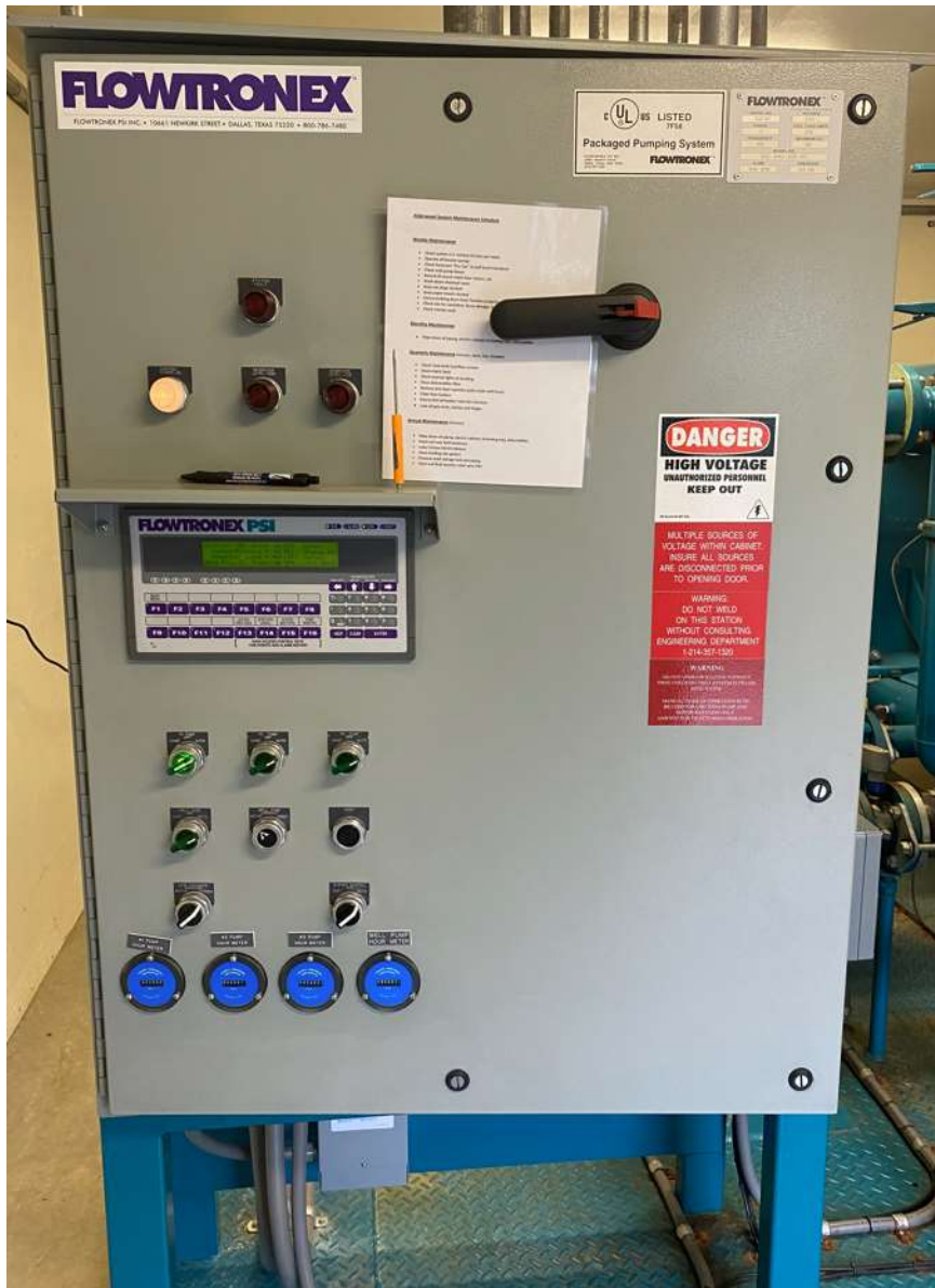
Existing Pump Control Panel: Replace internal backpanel assembly complete. Remove existing door devices and replace with new door skin and devices.
