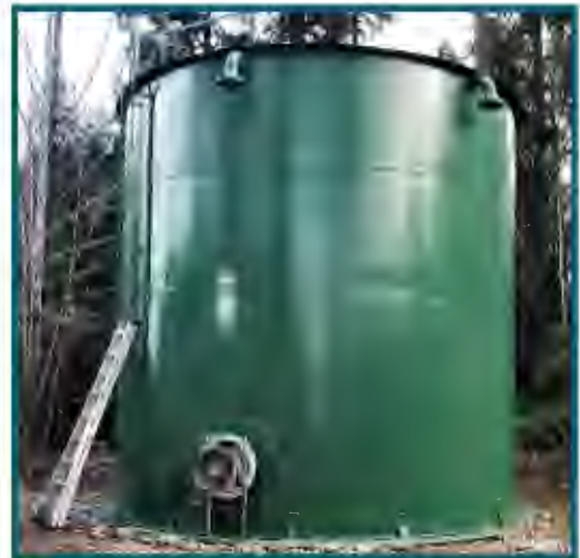
Tank Recoating Project
